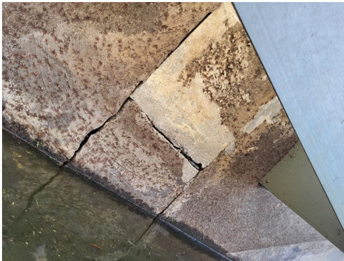
Photo showing cracks on south side of concrete structure below the weir.
