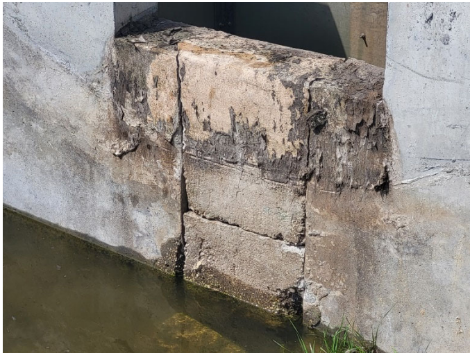
Photo showing cracks on south side of concrete structure below the weir.
